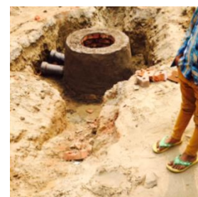
Sewerage works started in one of the communities
